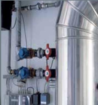
An EV250B solenoid valve, a great all-round valve, is the preferred choice for many manufacturers in applications with low differential pressures, such as heating systems. Its design not only allows for a wide pressure range, it also reduces noise and increases the lifetime of the system through water hammer dampening.
